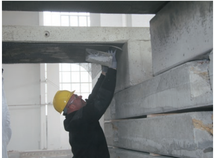
Fig. 3.5: Incorporation of textile in the fine concrete layer
