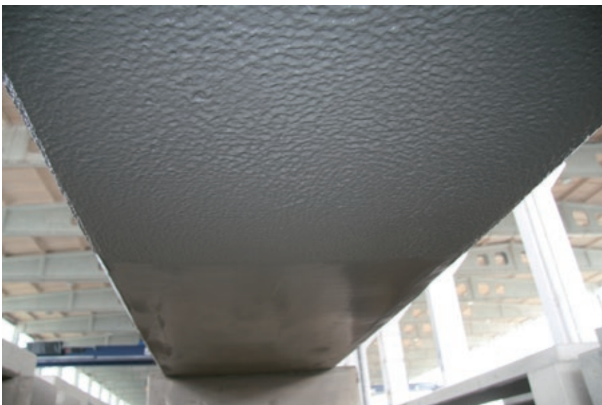
Fig. 3.9: Final layer – unprocessed in the foreground and already smoothed in the background.
