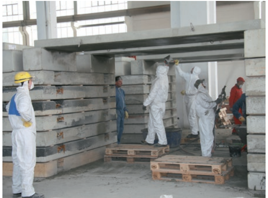
Fig. 3.8 Demonstration of simultaneous work process: In the background on the left: 2 workers incorporating the reinforcement layer. In the background to the right: Splashing of fine concrete for preparation for the next layer or the final layer of fine concrete.
