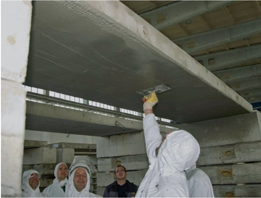
Fig. 3.8 Demonstration of simultaneous work process: In the background on the left: 2 workers incorporating the reinforcement layer. In the background to the right: Splashing of fine concrete for preparation for the next layer or the final layer of fine concrete.
