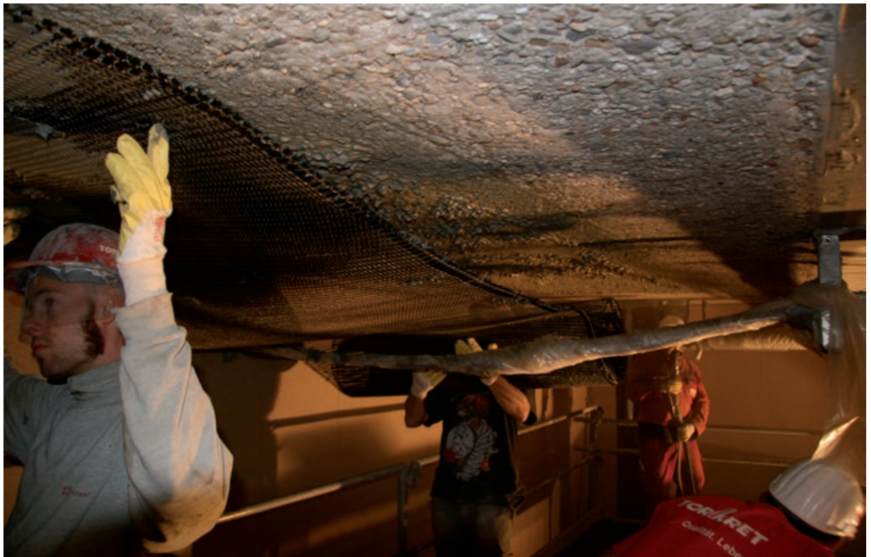
Textile concrete reinforcement Canyon Bicycles GmbH in Koblenz
