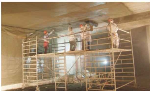
Reinforcement of a department store in Prague
