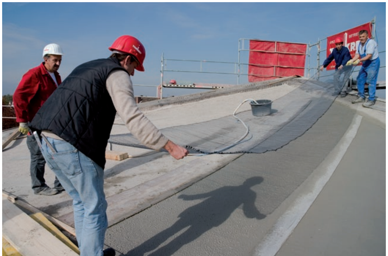
Reinforcement of a hypar shell roof in Schweinfurt
